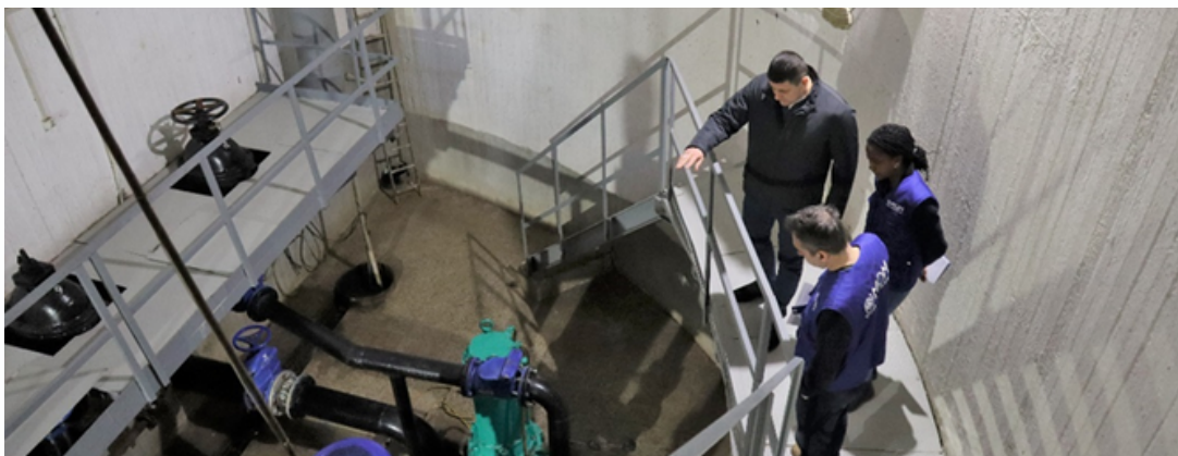
Replacing old pumps and equipment , Ukraine © IOM 2022
